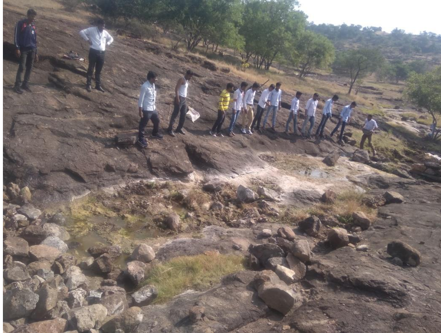
CCT Construction Work at Tandulner Tal. Rahuri Dist. Ahmednagar
